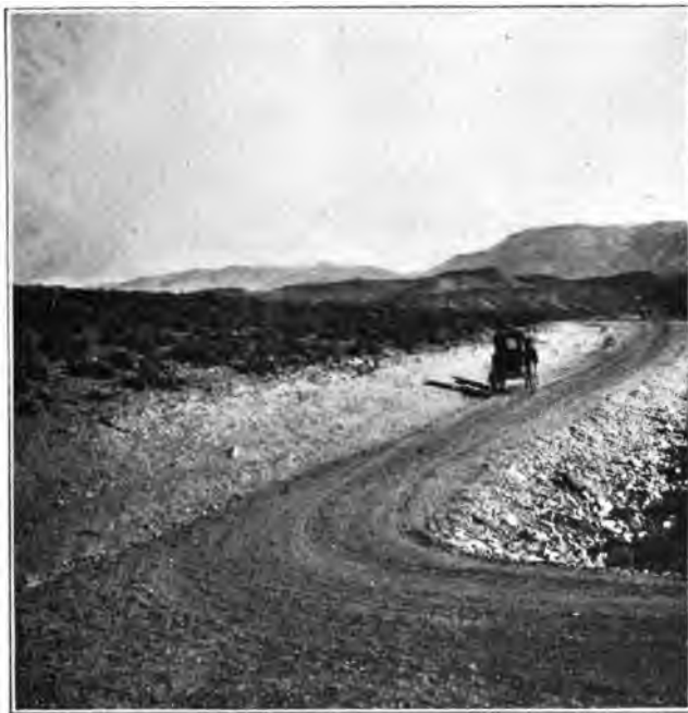
NEW STATE ROAD, PIUTE COUNTY.
